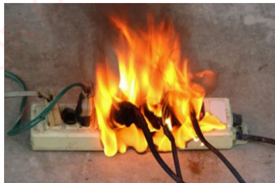
Figure 6.2: Electrical fire caused by power surges
